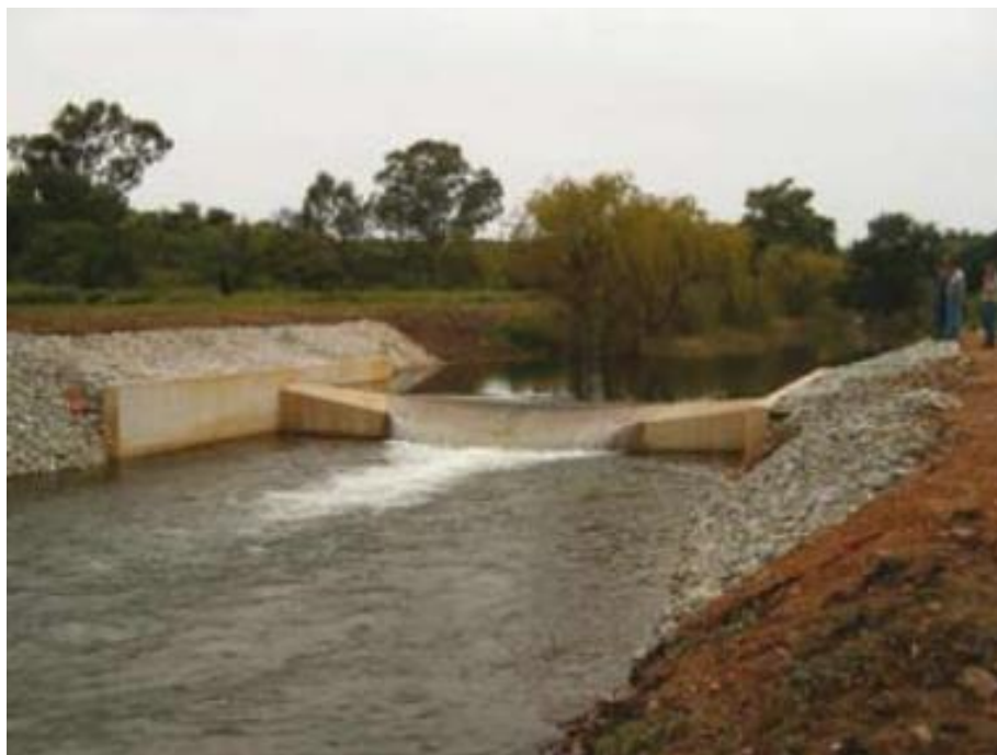
Figure 10: Example of a V-shape Crump weir in the Mooi River near Potchefstroom (North-West Province) (Wessels and Rooseboom, 2009).
