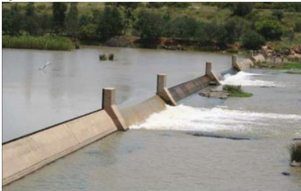
Figure 8: Example of a compound sharp-crested weir in the Vaal River downstream of Vaal Dam (Wessels and Rooseboom, 2009).
