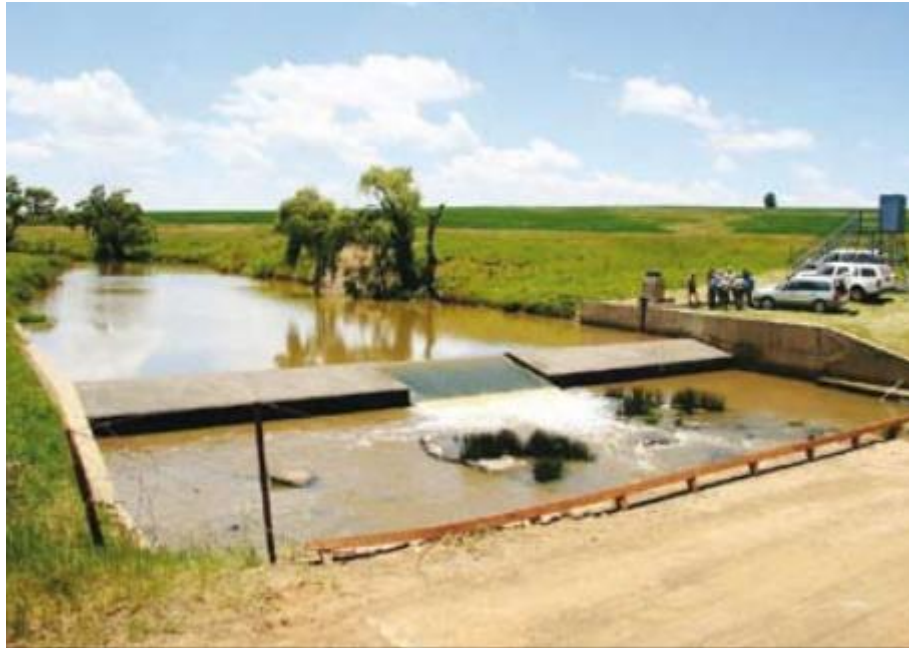
Figure 9: Example of a horizontal compound Crump weir without dividing walls in the Vaal River catchment (Mpumalanga) (Wessels and Rooseboom, 2009).
